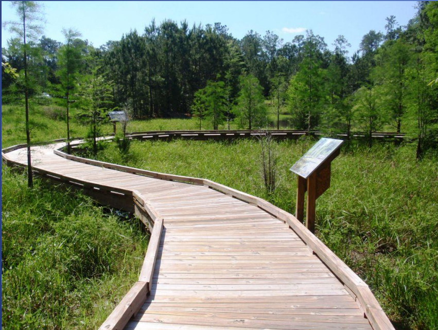
UF –Stormwater Ecological Enhancement Project (SEEP) An example of an enhanced basin
