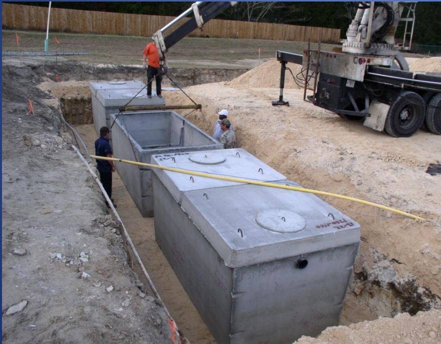
Fire Station 17 (Jonesville) - Storage tanks under parking lot for stormwater reuse
