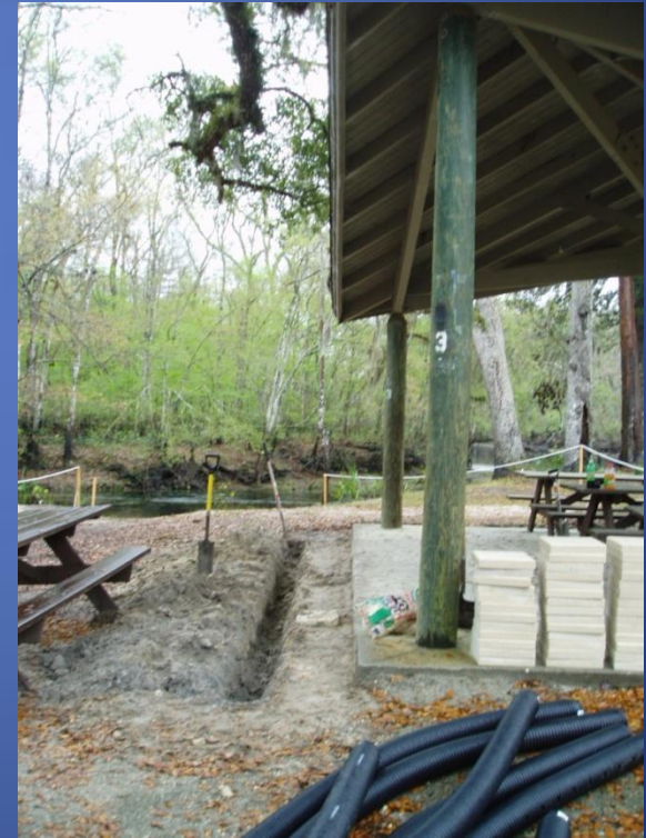
Infiltration trench at Poe Springs Park
